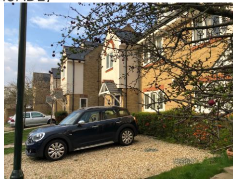
North Lane New Development
